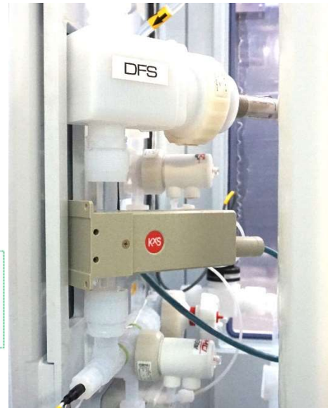
Fig.2 Integration of KxS Technologies inline refractive index monitor
